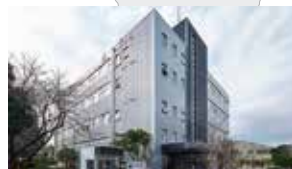
Hitachi Industrial Equipment Systems Co., Ltd. Sagami Works (Kanagawa, Japan)
