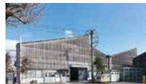
Hitachi Industrial Equipment Systems Co., Ltd. Rebuild & Engineering Center (Kanagawa, Japan)
