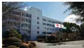
Hitachi Industrial Equipment Systems Co., Ltd. Tsuchiura Works (Ibaraki, Japan)
