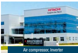
Air compressor, Inverter
