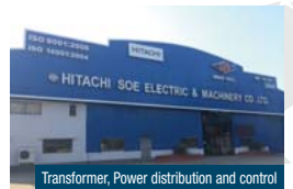
Transformer, Power distribution and control
